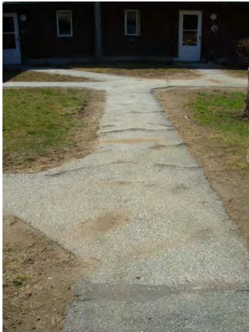
3. Sections of walkway cracking and heaving
