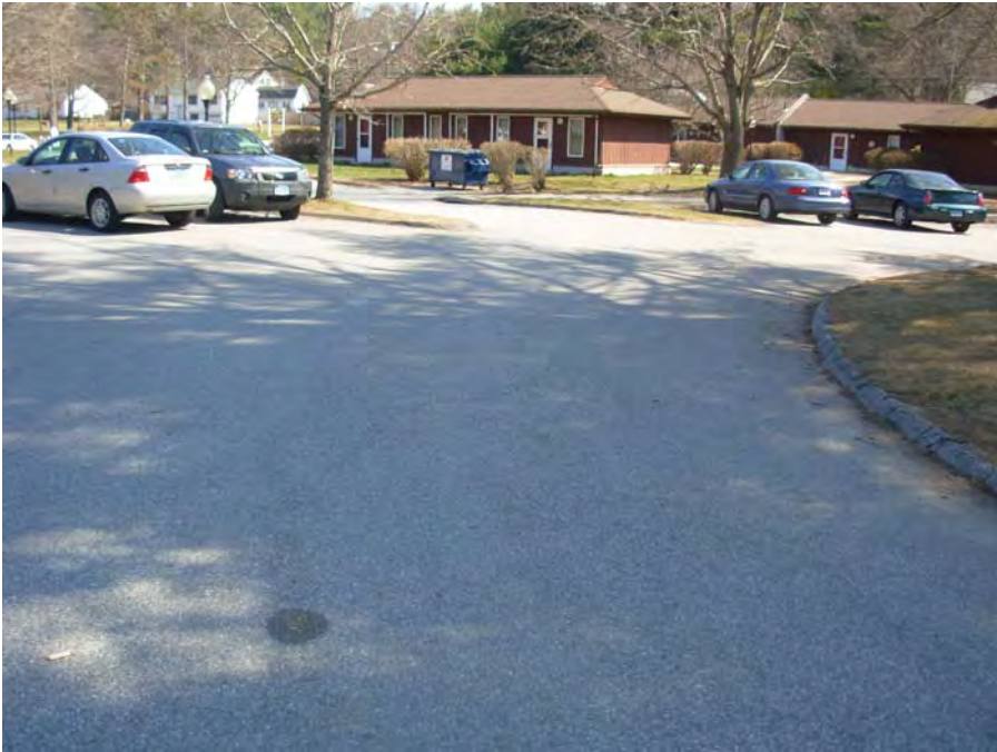
1. Typical parking area surfaces, minimal cracking
