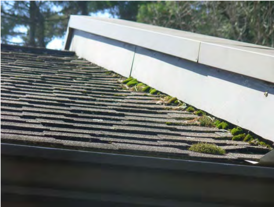
9. Spot shingle lifting and organic material building on roofing shingles
