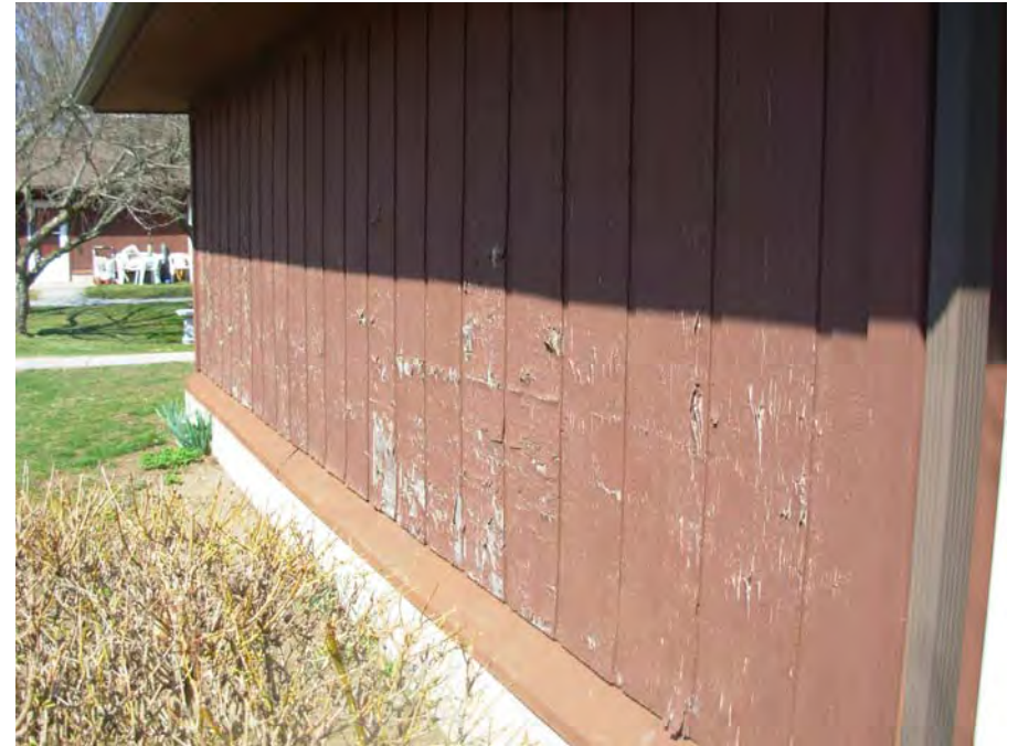
6. T-111 siding deterioration, to clad with vinyl siding
